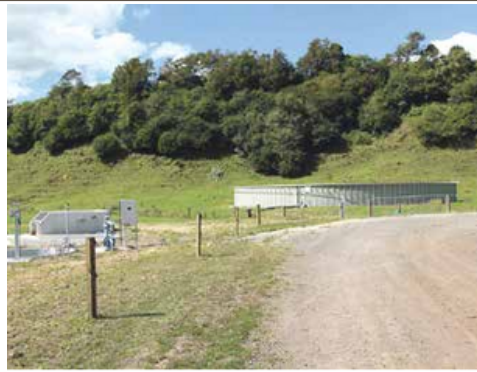
The new effluent system – sand traps, bunker and Kliptank.
